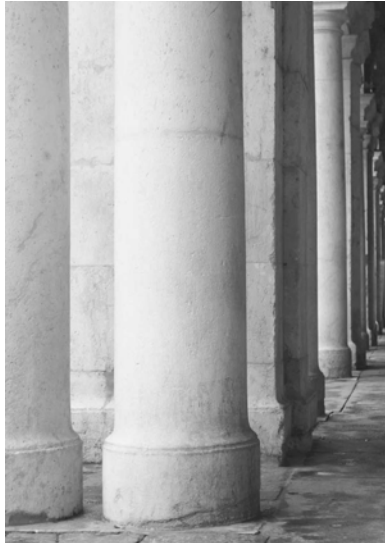
14 Andrea Palladio, the Basilica in Vicenza, detail of the bases on the ground level, 1549–1561.
