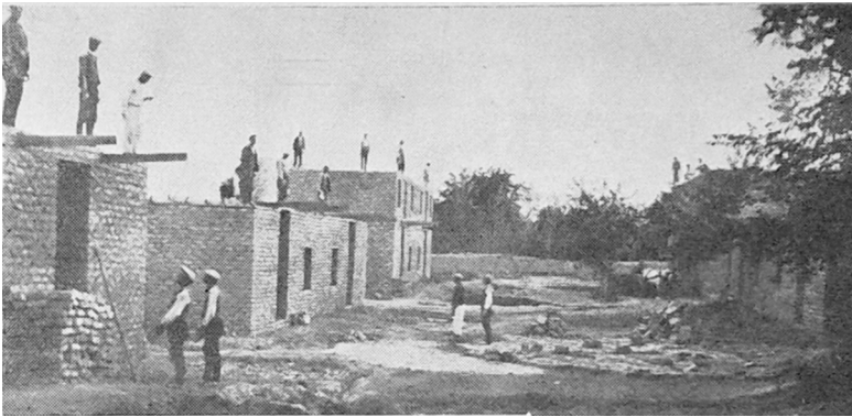
Figure 5.8. Settlement in Perçenç (Akçakiraz), built in 1935. 83
