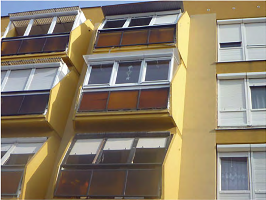
Figure 1: Informal balcony enclosures.
