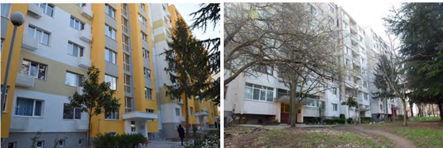
Figure 4: Retrofit of multifamily housing in the housing estates of Burgas.
