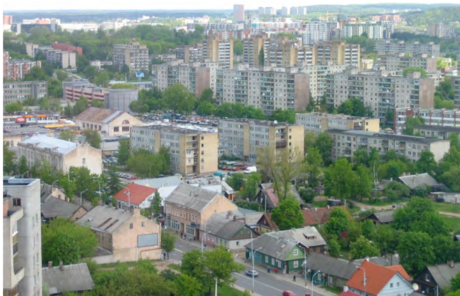
Figure 1: Prefabricated and traditional housing in Vilnius.
