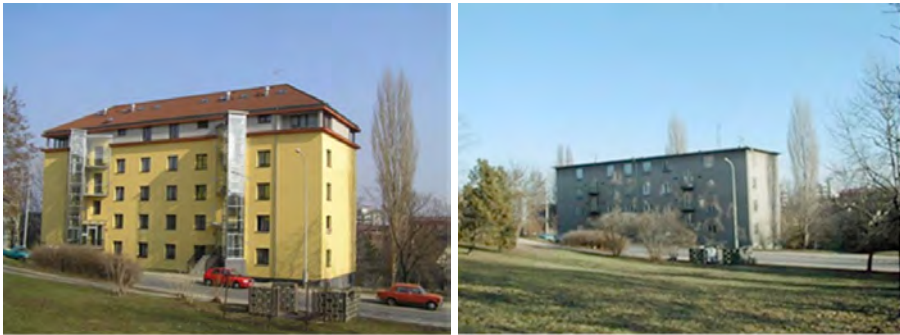
Figures 2.1 + 2.2: Renovation of prefabricated housing in Czech Republic and Hungary.
