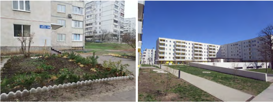
Figure 7: Parking garage beneath a yard after renovation, Dresden, Germany.
