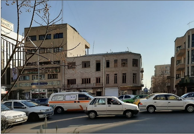
Figure 42: Examples of beautified facades in Enghelab Street
