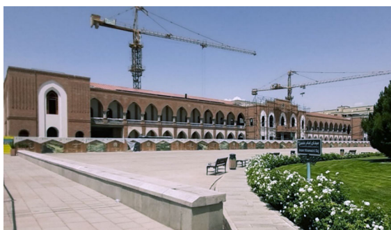
Figure 53: The ongoing reconstruction project of the Baladiyeh
