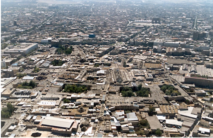
Figure 24: The preserved roofscape of Tabriz Bazaar, the 1990s
