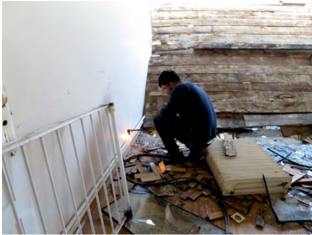
Figure 5.7: Cutting metal pipes 10
