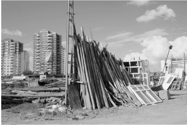
Figure 6.17: The beams from old vernacular houses are used for roof structures
