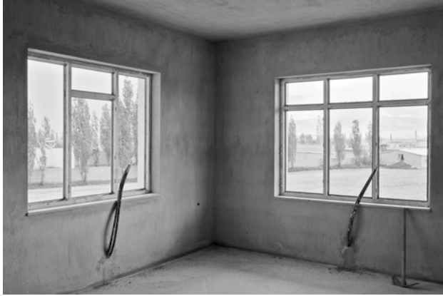
Figure 7.7: PVC window frames from Istanbul in Yazıhüyük
