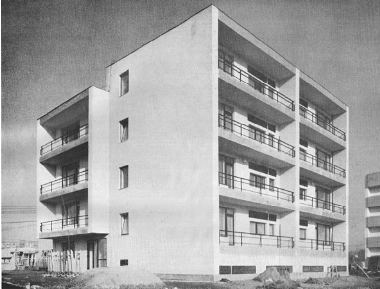
Figure 1: Apartment house, Budapest 1961. Architect: Olga Mináry (1929-2000). Mináry received the Ybl Prize for this building in 1964. Source: Magyar Építőművészet 1961, 1, 11.
