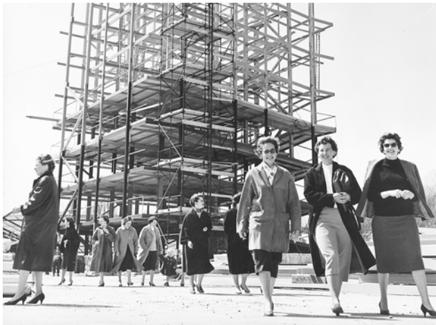
Figure 2: Women architects visiting the SAFFA Tower construction site, 1958. Source: Bequest Annemarie und Hans Hubacher (gta Archives, ETH Zürich).
