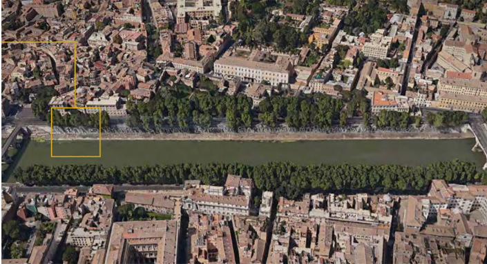
Figure 10. Detail of the intervention.
