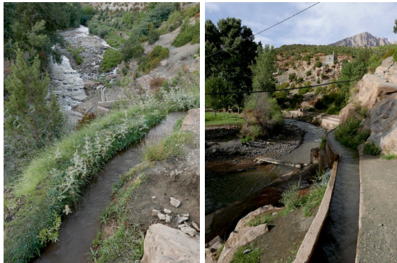
Figure 12 & 13: Irrigation channels on different levels next to the river
