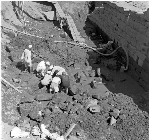
Figure 17. Chevrier's 1940s excavation in front of the western tribune. The two mooring rope loops in course four and five are visible. The pump is located at c.70.50 m, five masonry courses below the stone loops (Photo no. 6112 ©CFEETK).
