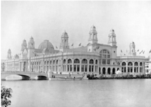
Figure 1: Electricity Building, World's Columbian Exposition, Chicago 1893.
