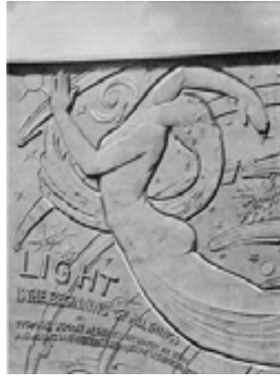
Figure 4: Bas-Relief Panel "Light" at the Electrical Building, Chicago World's Fair, 1933.
