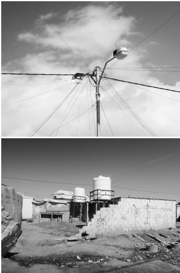
A lighting pole, tapped into by multiple families in Zaatari camp A dismantled communal latrine in the old camp
