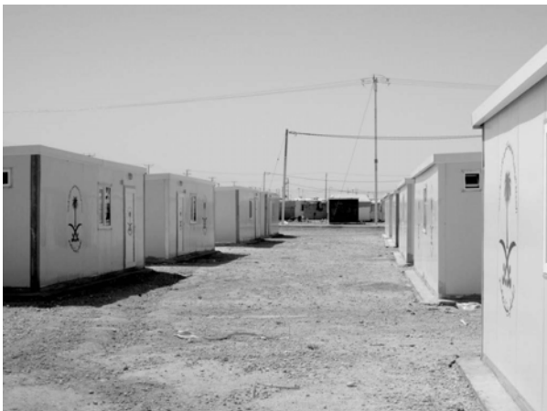
The Saudi fixed caravans, with a built-in kitchenette and bathroom/toilet
