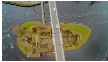
Fig. 11b: Ruins of Kajaani Castle with modern bridge (built in 1937).
