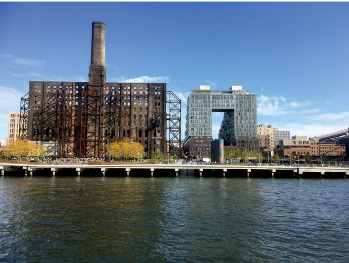
Fig. 3: The New York waterfront at Williamsburg, Brooklyn, with Domino's Factory redevelopment. Image by Lieven Ameel. October 2019
