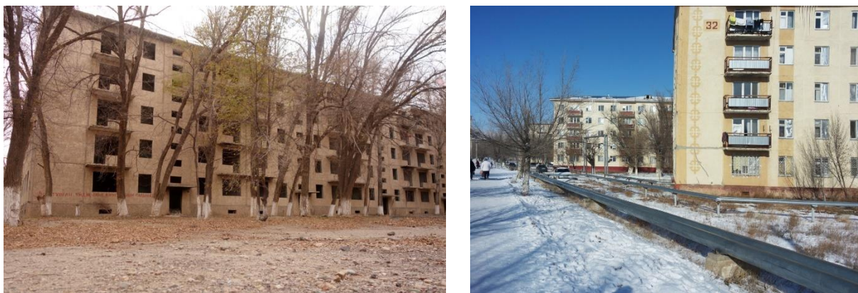
Figure 2: The residential houses of the 1st city district repaired within the state programme, November 2018
