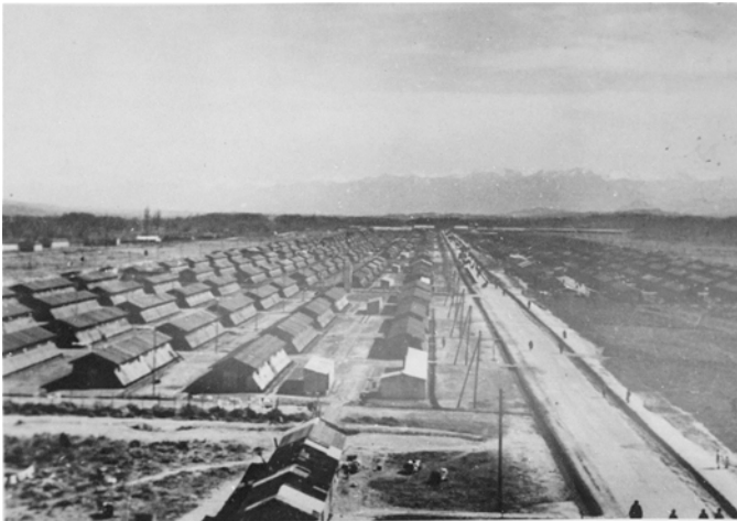
Figure 2: Photo of Gurs
