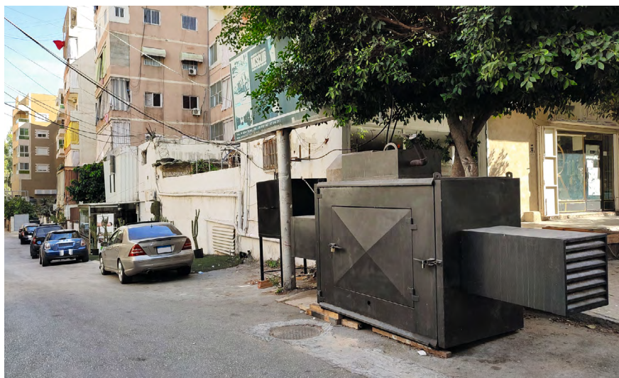
A private diesel generator at ground-level for alternative power supply at a street corner of Tyre, southern Lebanon. It runs and emits exhaust fumes for about 18 hours a day. Photo: Karim Eid-Sabbagh
