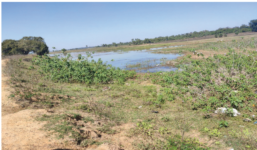
Figure 3.4: Tank in Nagampet village (before renovation) in Mancherial district
