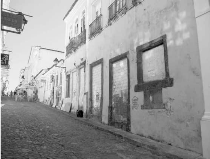
Figure 2: Facadism and gentrification. Houses in the Pelourinho district (Photo: G. Vinken 2014)
