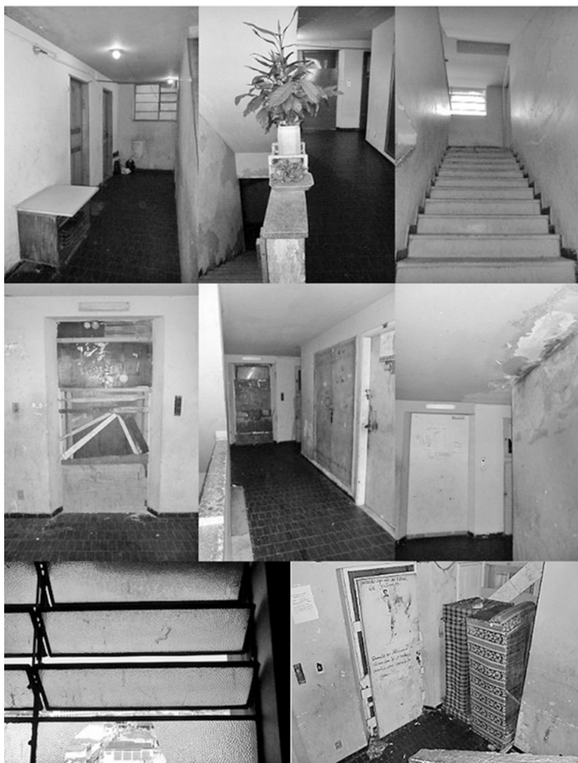
Figure 8: Corridors and stairways of the building 27
