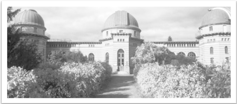
Figure 4: Michelson House. The former Astrophysical Observatory, now the headquarters of the Potsdam Institute. Source: Own photo
