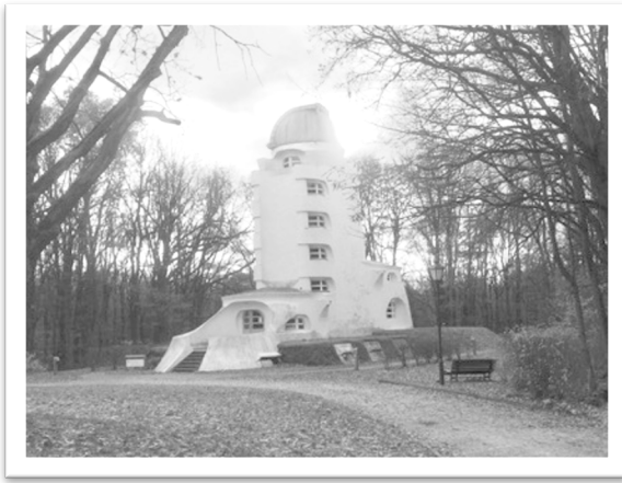
Figure 8: Einstein Tower. Source: own photo
