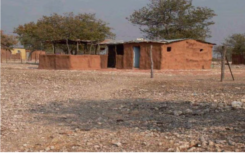
Figure 5: House built with local materials
