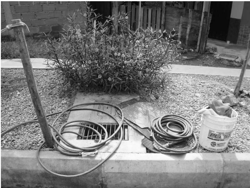
Figure 2: Technical interventions in carwash sites implemented by EPM: Installment of water meters, construction of drainage systems and provision of hoses. (Marcela López 2017).
