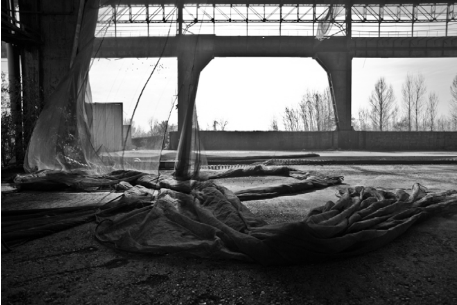
Figure 5: Falck Concordia inside view (Photo: U. Gillio 2015)
