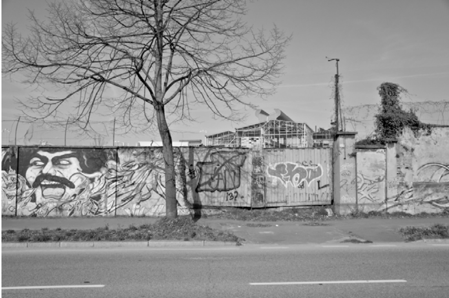
Figure 11: Street art on Viale Italia. The Unione plant in the background, with its pincer-shaped roof, rebuilt in the 1950s and still visible, is a Falck landmark (Photo: U. Gillio 2015)
