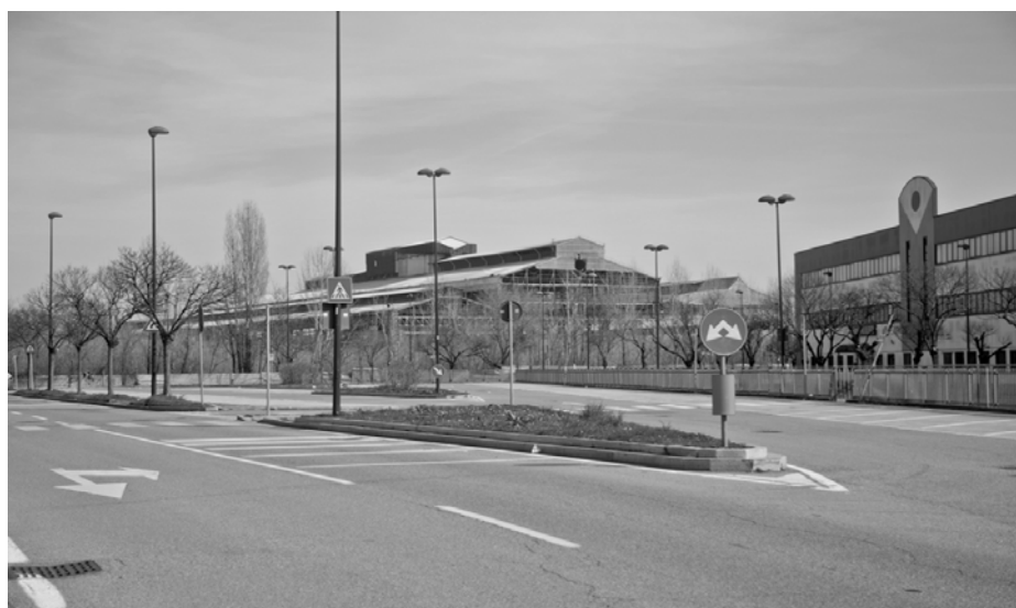
Figure 1: Falck Concordia plant viewed from Viale Italia, Falck area's main longitudinal axis, in Sesto San Giovanni (Photo: U. Gillio 2015)
