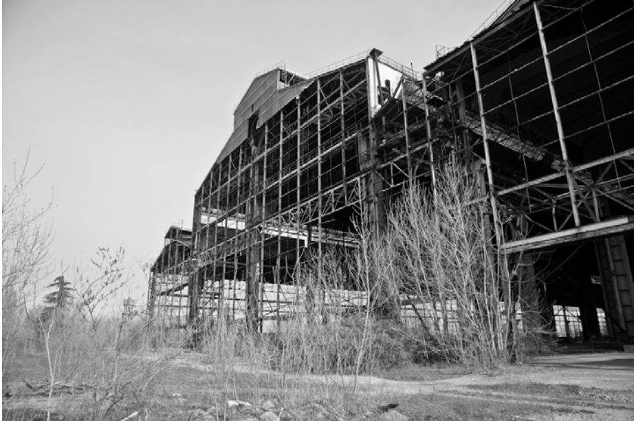
Figure 2: Falck Concordia plant viewed from the outside (Photo: U. Gillio 2015)
