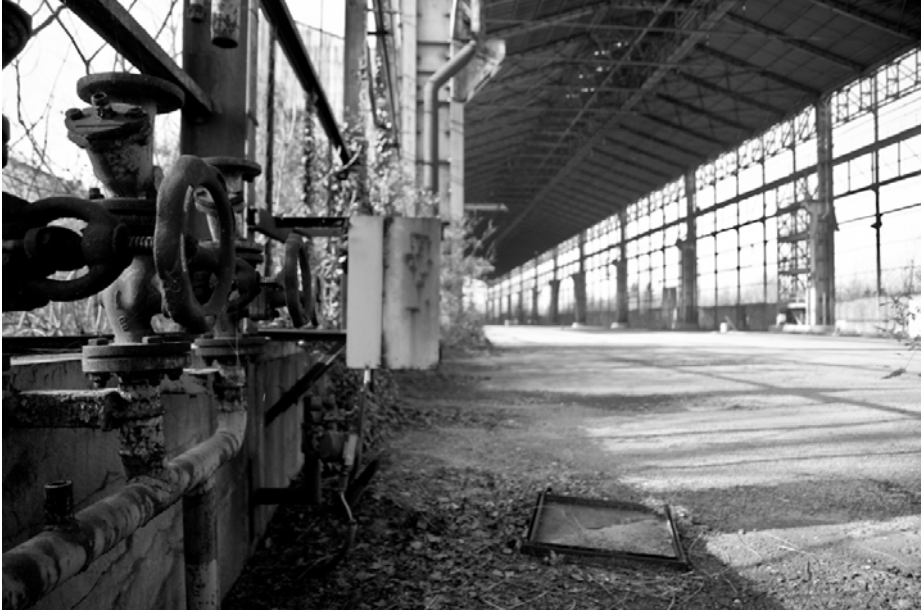
Figure 4: Falck Concordia inside view (Photo: U. Gillio 2015)
