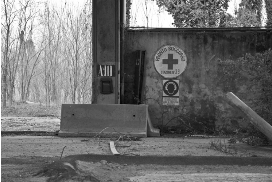
Figure 8: Rusty production signs, still imparting instructions and orders (Photo: U. Gillio 2015)
