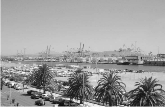
Fig. 4: Parts of the Llano Amarillo area with view to some port facilities in the back (photo: Carolin Alfonso)
