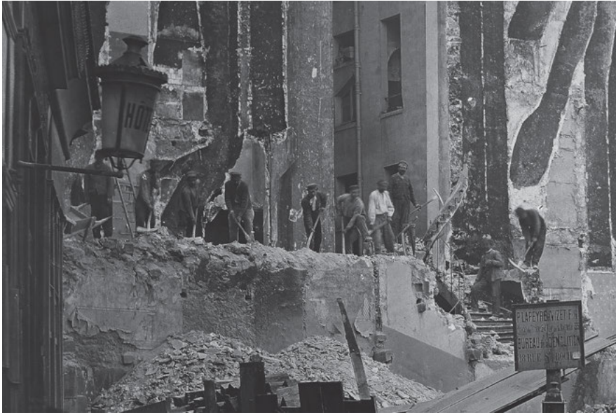
Fig. 3: Construction work to open up the Avenue de l'Opéra (1870–77) photograph by Charles Marville (excerpt).
