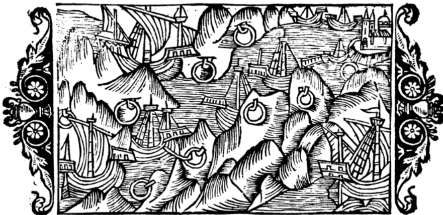
Figure 5.1: Mooring rings along the Norwegian coast near Bergen, from Olaus Magnus, Historia de gentibus septentrionalibus (1555). Similar constructions were in use on the North Atlantic islands.
