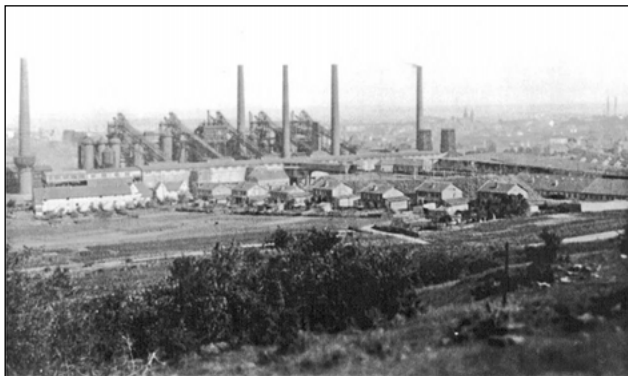
Figure 5: The estate Kazeberg beside the technical installations of the Usine Terre Rouge in the late 1920s (Photo: private)
