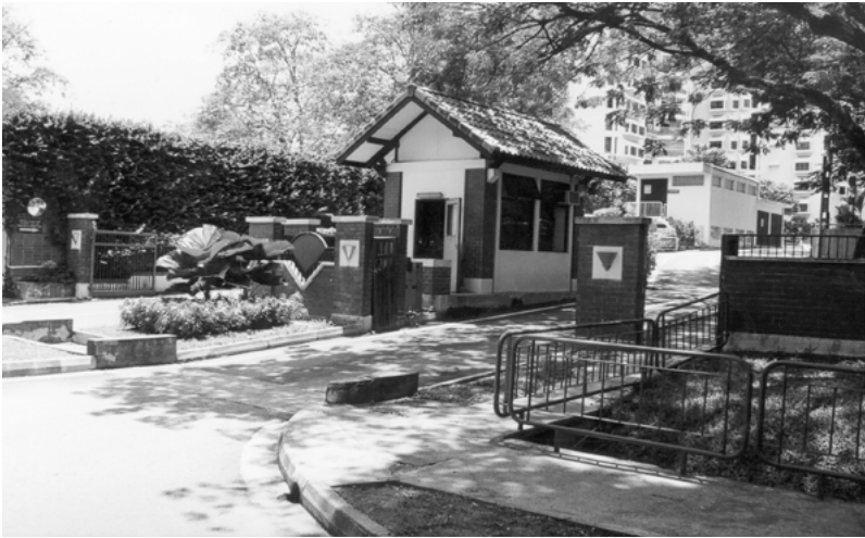
Figure 4: Gate of a condominium (Photo: © Lars Meier)
