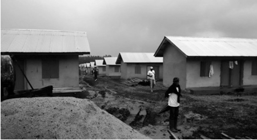
Figure 7.1: A new CDC camp under construction: laborer camps. Notice the well-aligned buildings.
