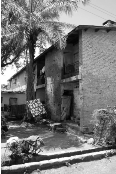
Figure 3.9: Two-story OCA houses erected in the “experimental site” in the Kamalondo neighborhood, situation anno 2010. Source: photograph by Céline Fenaux, 2010.
