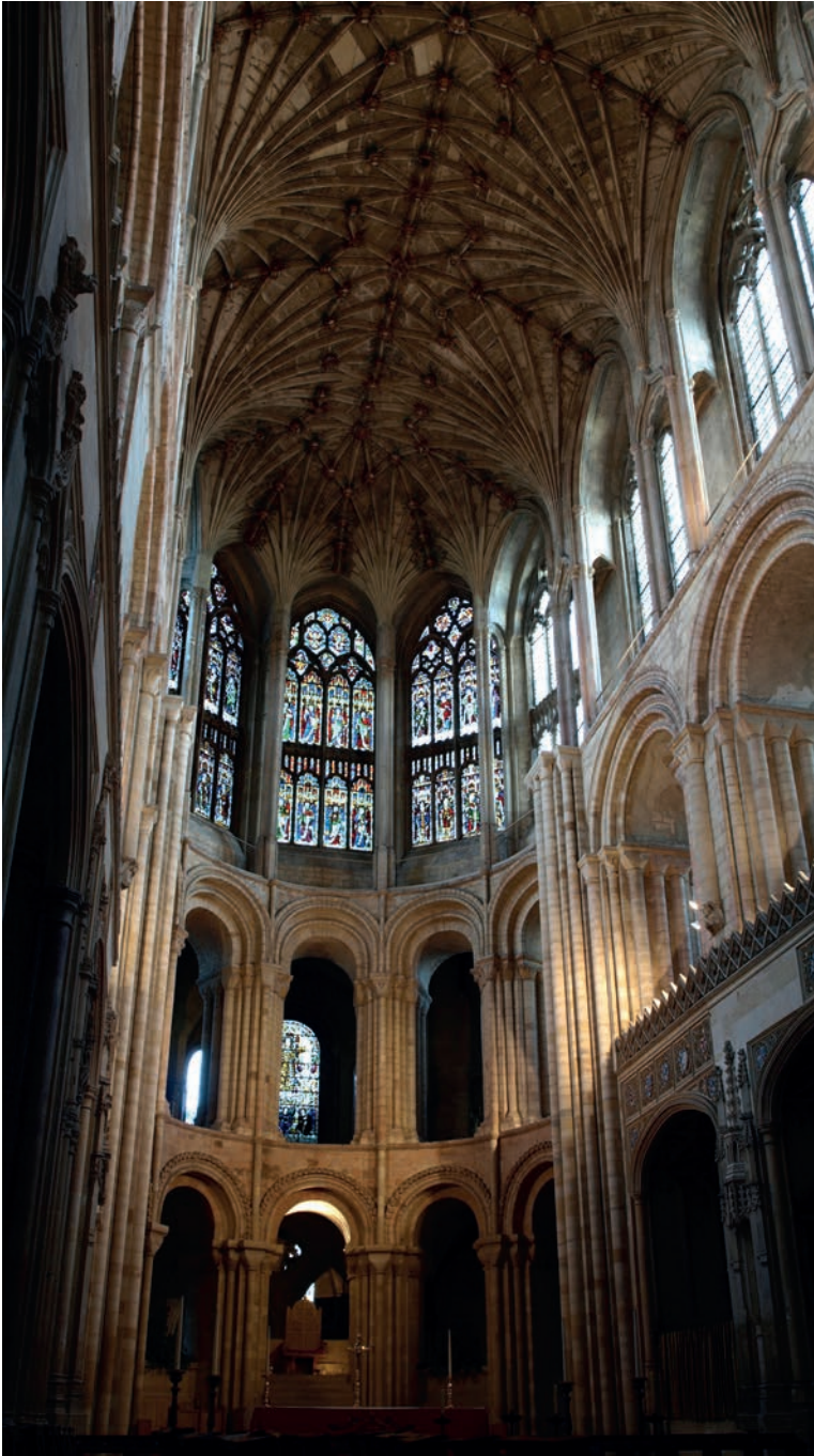
Figure 1: The presbytery of Norwich Cathedral. Although the current clerestory was remodelled in the 15th century, the disjuncture between Romanesque and gothic architecture above the first floor is a direct result of damage caused on St Maur(us)'s Day 1362. (Photograph by the author).
