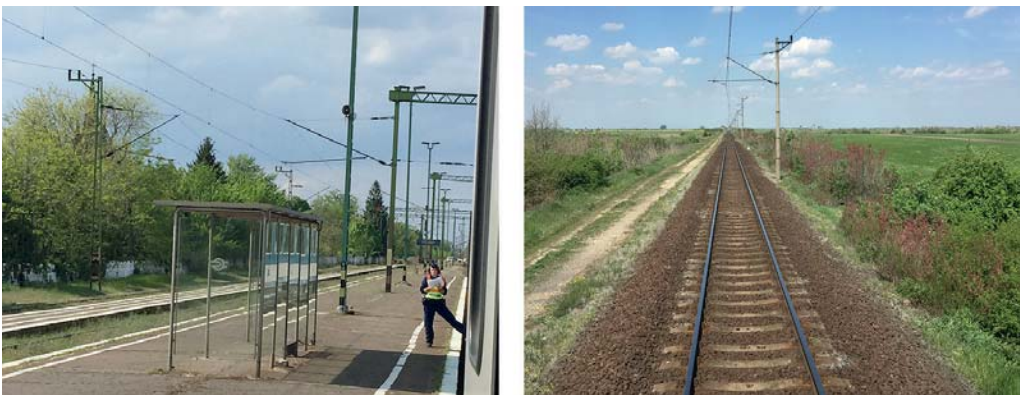
Fig. 2: Corridor capacity and performance challenges Budapest–Beograd: waiting times at borders (e.g. Kelebia, Hungary, left) and single-track infrastructure produce travel time losses / Source: Author
