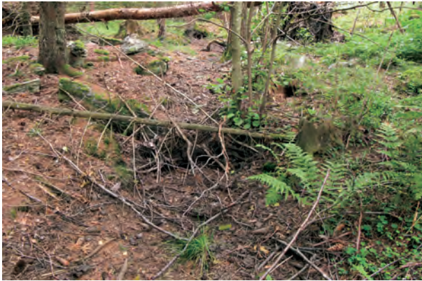
Fig. 36 It is difficult to imagine that this hidden stone heap is a dam to provide water power for the bellows at the smithy of a shipyard. Björkö, Dalsland. (Photo: Christer Westerdahl)
