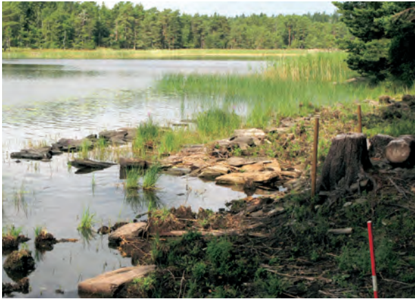
Fig. 51. Remains of a stone and timber caisson, krängkista , for careening ships at Björkö, Dalsland. (Photo: Christer Westerdahl, 2007)
