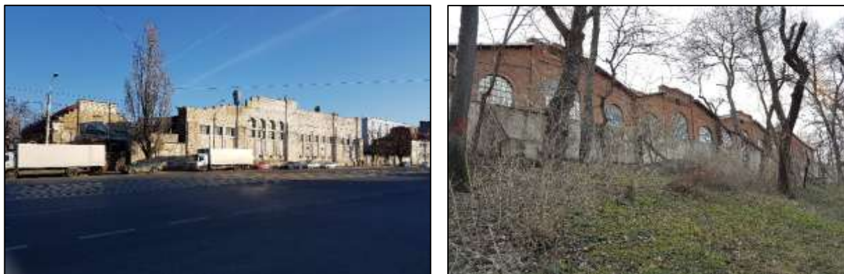
Figure 14 and 15. Buildings of the old E. Wolff S.A.R factory
