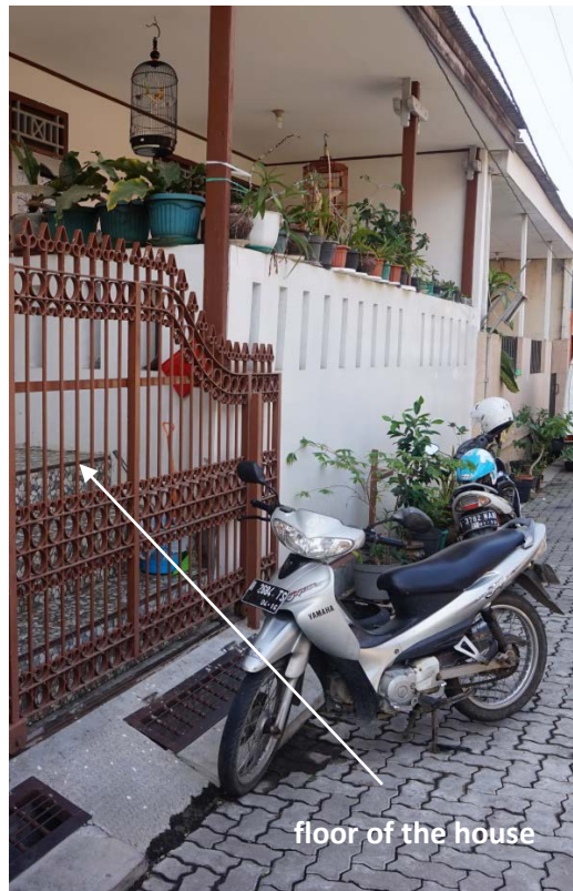
Picture 1: House in Kel. Panggung Lor whose floor had been lifted for 3m in total. (Picture: Ziegelmayer 2015)
