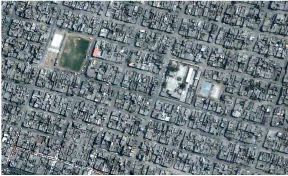
Figure 3. The streets in the Comás squatter community in Lima, Peru, are 10-meters-wide and take up 25% of the area. A 160m 2 house there now costs $180,000. Source: Google Earth.
