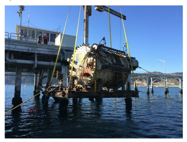
Image Attribute: Pulling out of Natick Prototype (Phase 1) from the shallow waters off California after 105 days of feasibility testing. / Source: Microsoft
