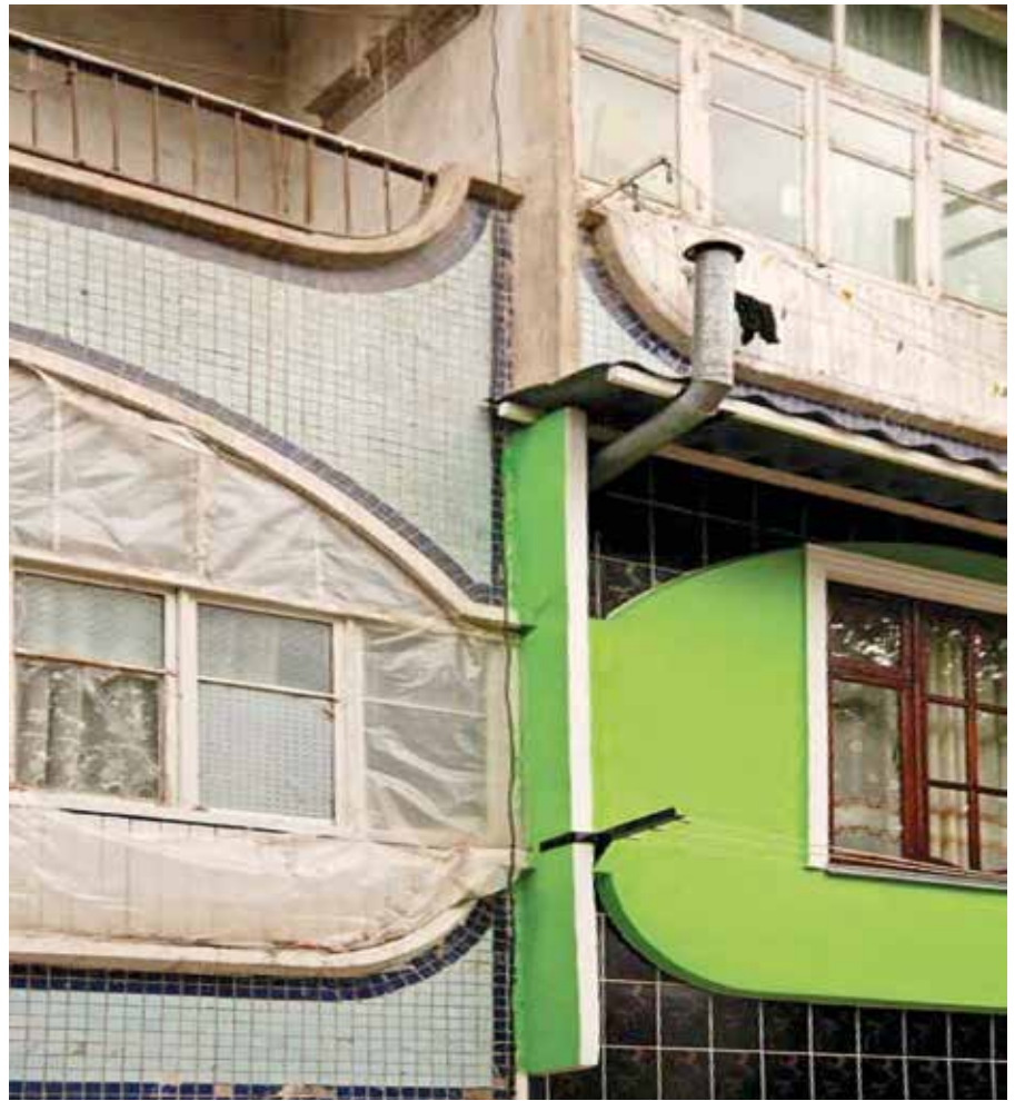
Photograph 2: Balcony enclosures reflect the owners' resources, 2010 (Wladimir Sgibnev)
