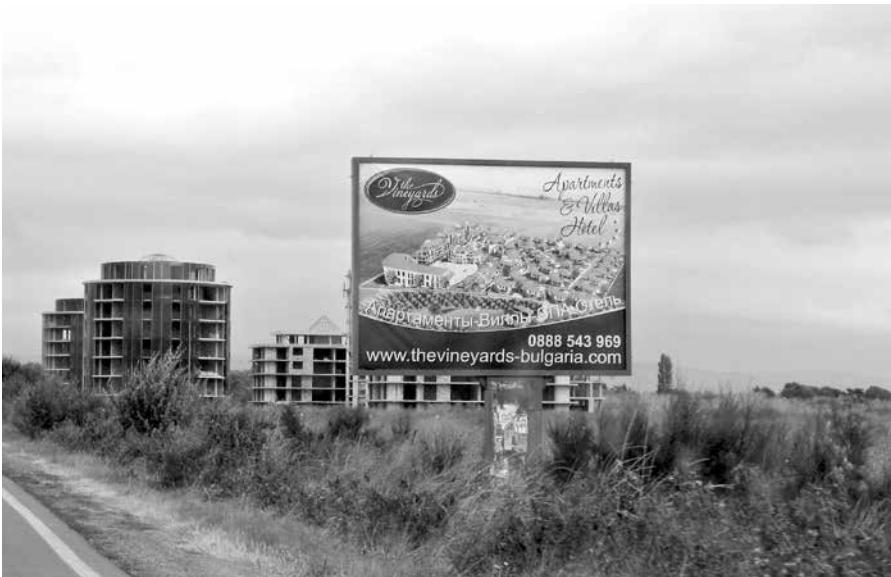
Photograph 9: Sunny Beach: new construction of apartment complexes, 2010 (Anke Hagemann)
