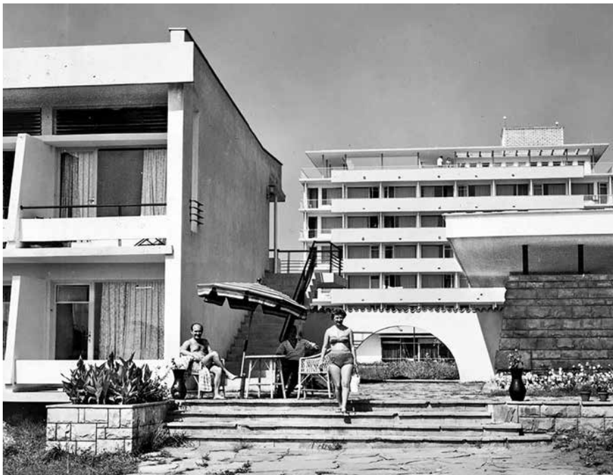
Photograph 2: Sunny Beach resort: modernist hotels in the early 1960s Source: Lost Bulgaria ( www.lostbulgaria.com )
