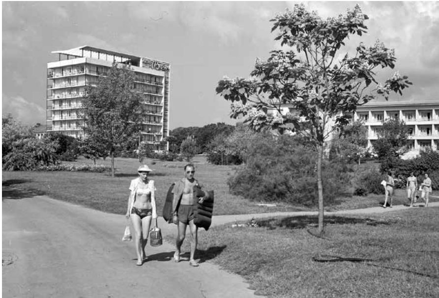
Photograph 1: Druzhba resort: first (right) and second (left) generation hotels in generous parkland, 1964 Source: BTA (Bulgarian News Agency)
