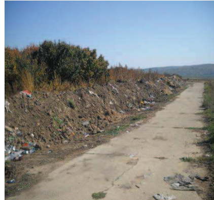
Fig.7 - Closed rural landfill – soil covered , uncompact, negative model, Bozieni commune, September 2009
