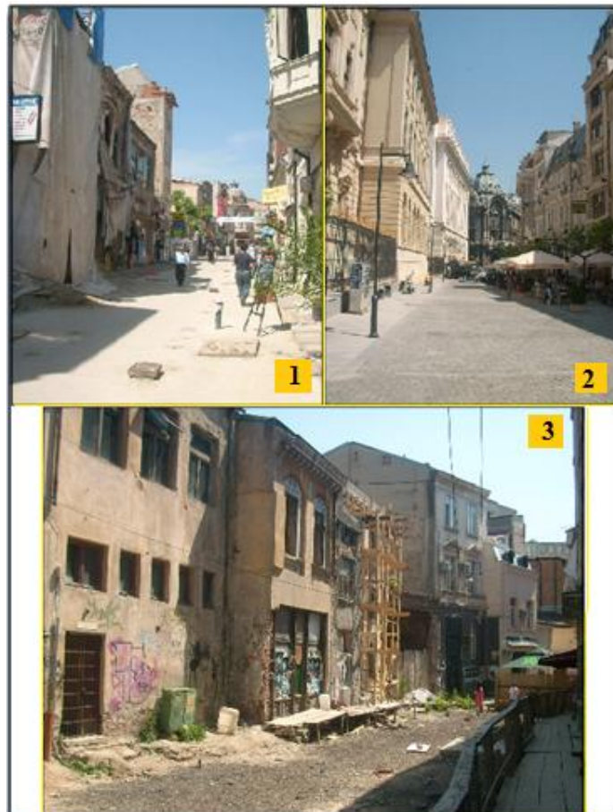
Image 1. Restoring the old center of Bucharest (Onea D. 2010) (1. Lipscani Street – 2. Smârdan Street – 3. Gabroveni Street)
