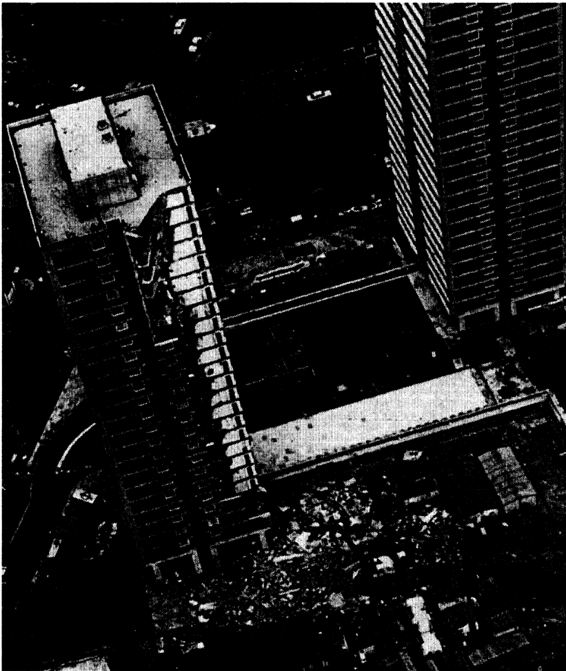
FIGURE 4 The collapsed south-east corner of Ronan Point, following the gas explosion. (Source: H. Griffiths et al. , Report of the inquiry into the collapse of flats at Ronan Point, Canning Town , Ministry of Housing and Local Government, 1968.)
