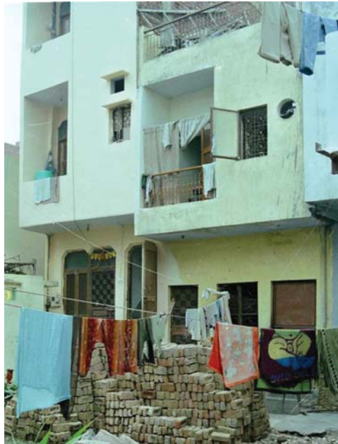
FIGURE 6 Sharda's two-storied house with steel-framed windows and doors. (Photo: Author, 2002.)
