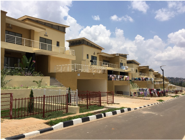
Figure 57. The Umudugudu Kigali Vision: Twin houses; front yard. Photograph by Manlio Michieletto.
