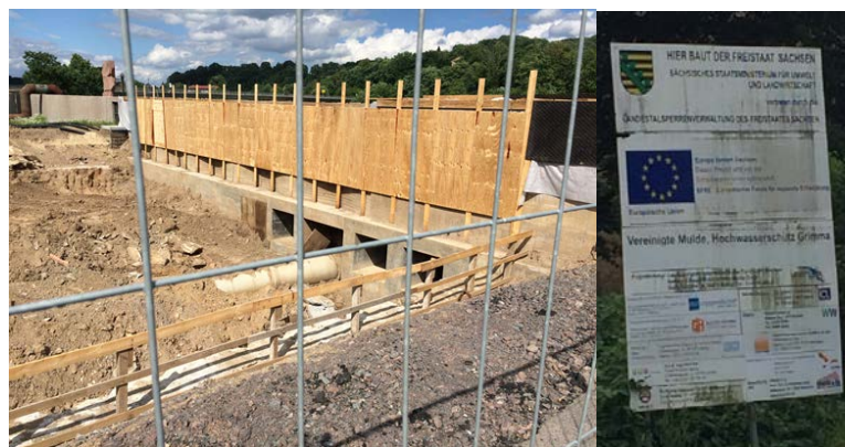
Figure 31 Floodwall, project 4, under construction (June 2017)
