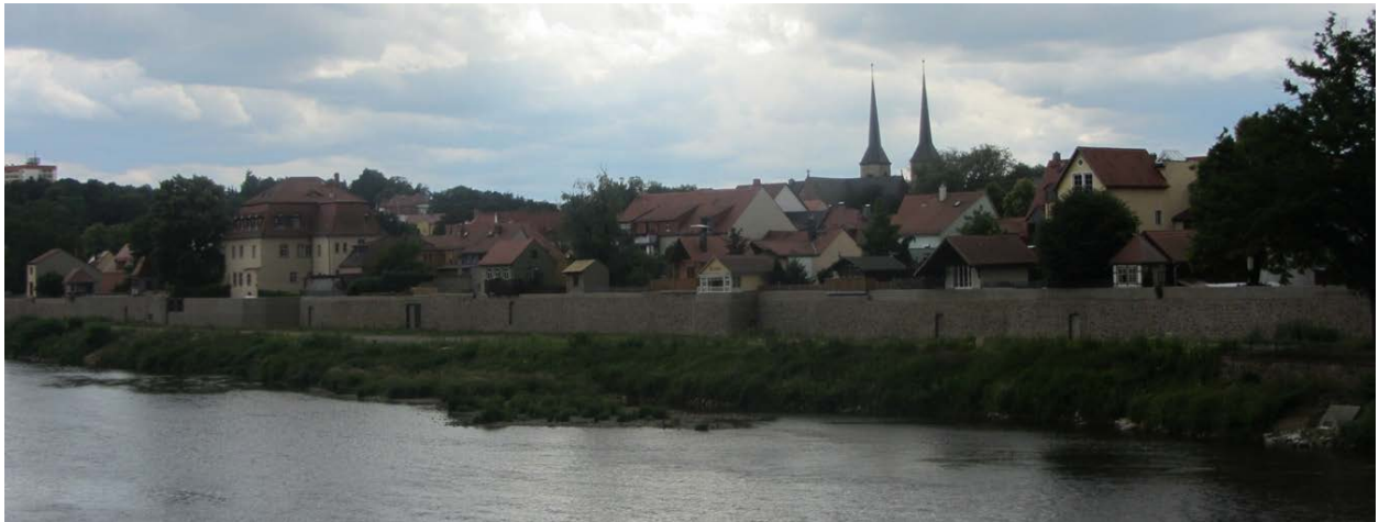
Figure 33 New floodwall, photo taken across the Mulde River by the authors (June 2017)
