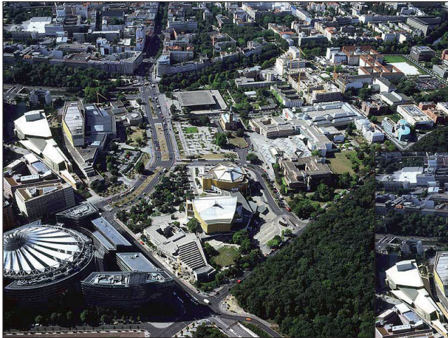
Aerial photo (view from north)
